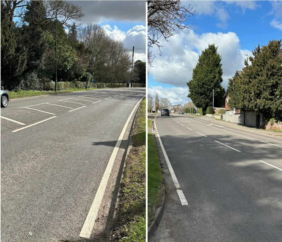
A county town road in the West Midlands Treated local road (surface dressing and encapsulation).
